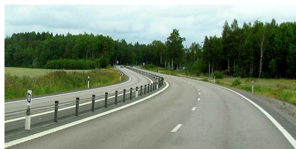
A 2+1 road with cable barriers.
